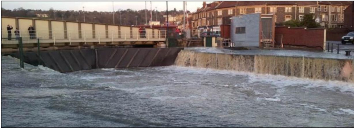
Figure 15 - Water shown overtopping the Junction Lock stop gates into the Floating Harbour
